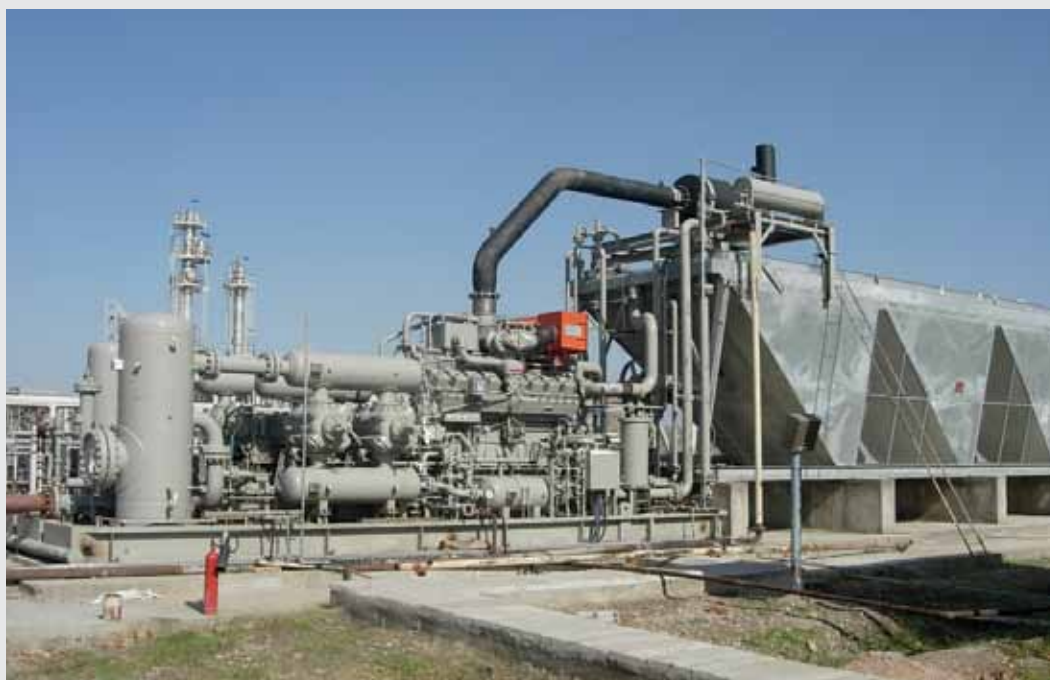
Gas compression recently installed at Chanda field
