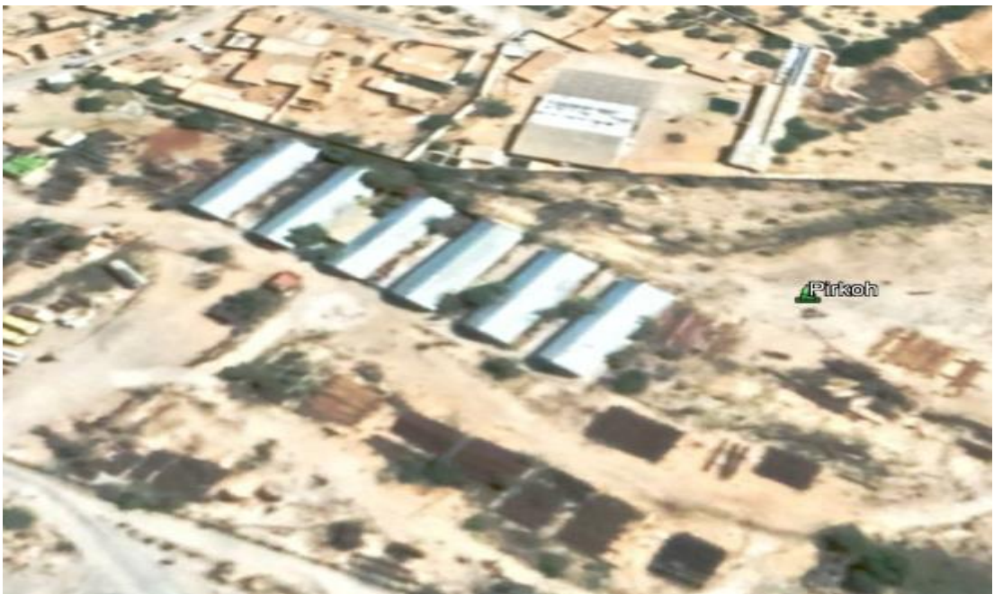
Pirkoh Gas Processing Facility
