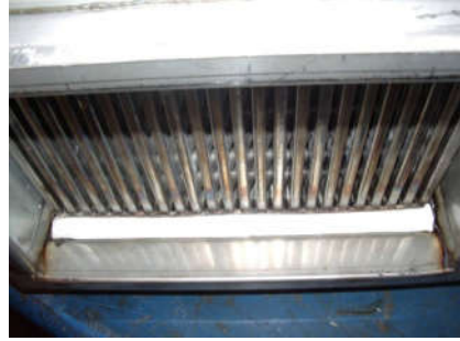
Figure 14: triangular PTFE cord installed in the groove of the column liner
