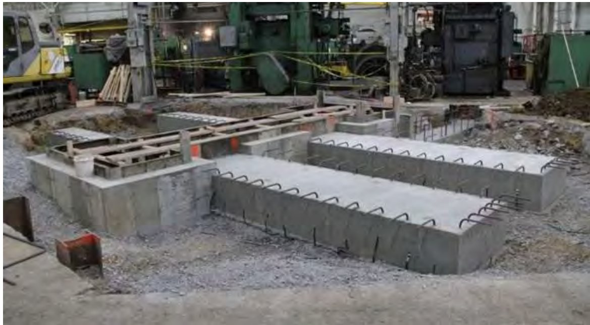
Figure 2.3 Typical machine foundation
