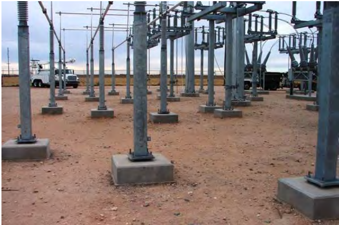
Figure 2.5 Typical foundation type for substations
