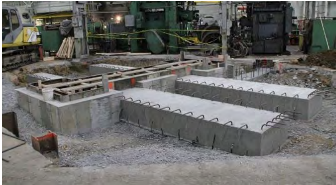
Figure 2.3 Typical machine foundation
