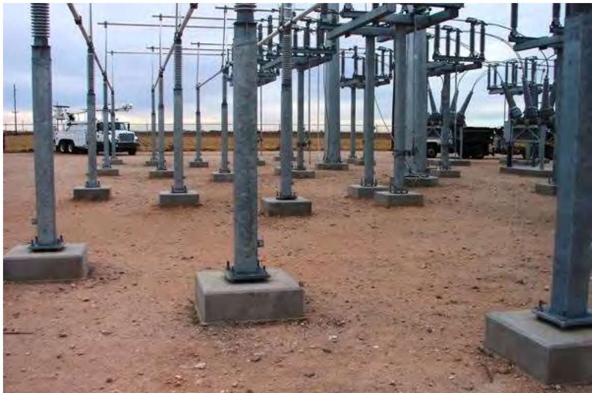
Figure 2.5 Typical foundation type for substations
