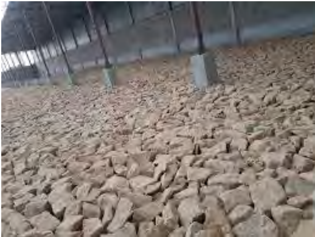
Figure 2.10 Stone soling work
