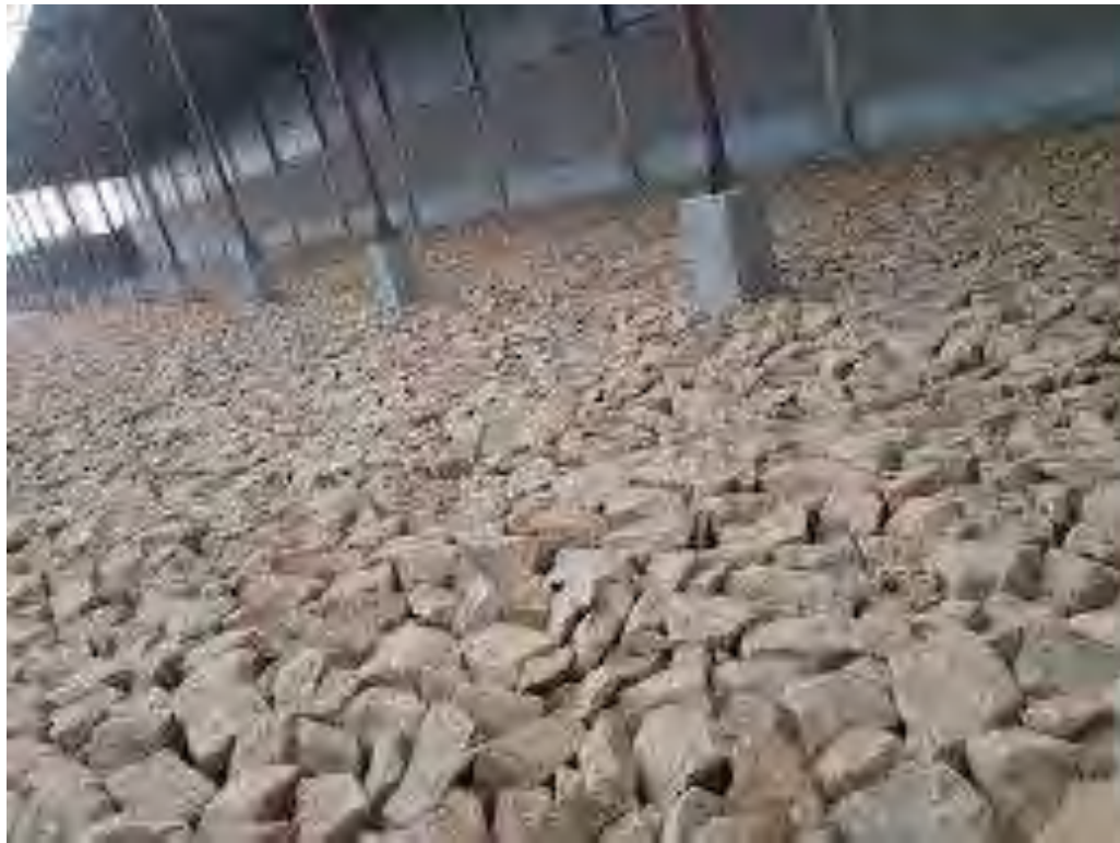
Figure 2.10 Stone soling work
