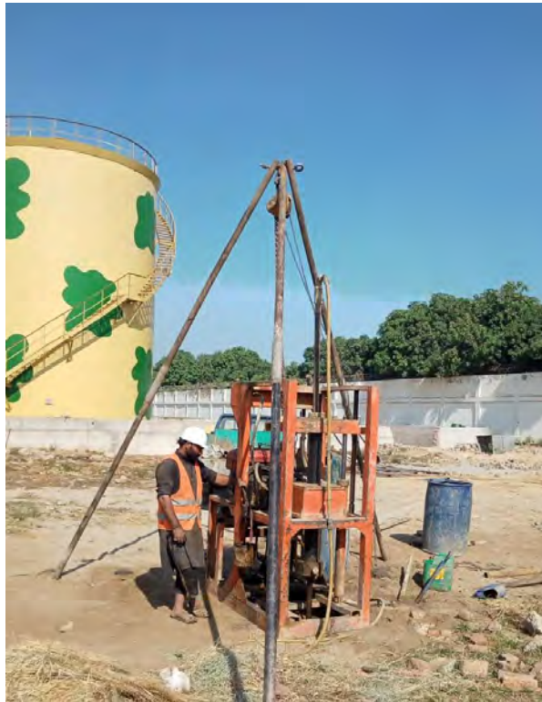
Figure 3.1 Straight rotary drilling machine
